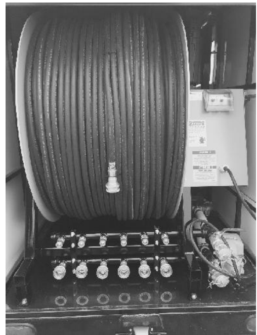
2 - GTS 300 Central Mobile Enclosure (back view)
