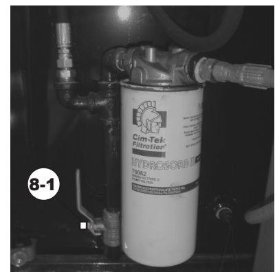
8 - fuel supply valve and filter
