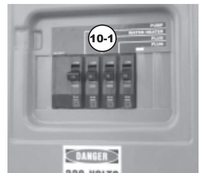
10 - 600 GTS breaker box
