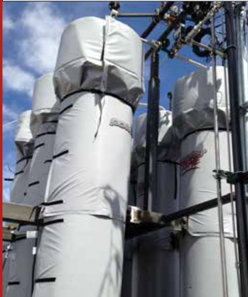
Processing Tank Heater
